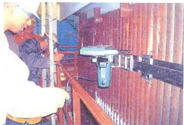
Boiler wall cutting
